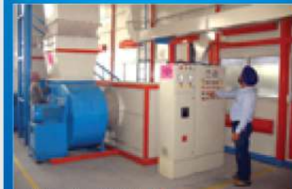
Inside View of Busduct Production
