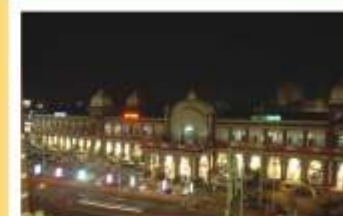
Egmore Railway Station, Chennai (External View)
